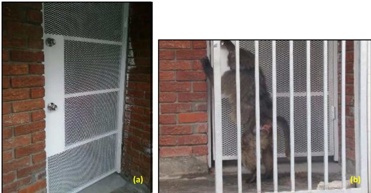
Figure 6: (a) Double door knobs at the bin bay cage. (b) Alpha female attempting to open the door by twisting only one door knob.
